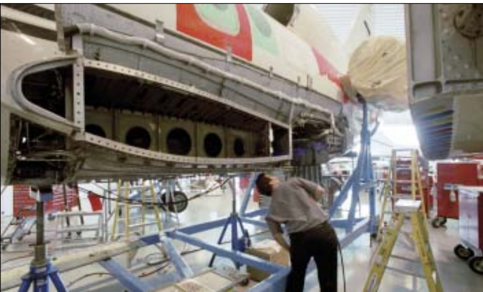
The Duncan Aviation Structures Team removes a wing from a Falcon 50 in order to repair corrosion found during an inspection.
