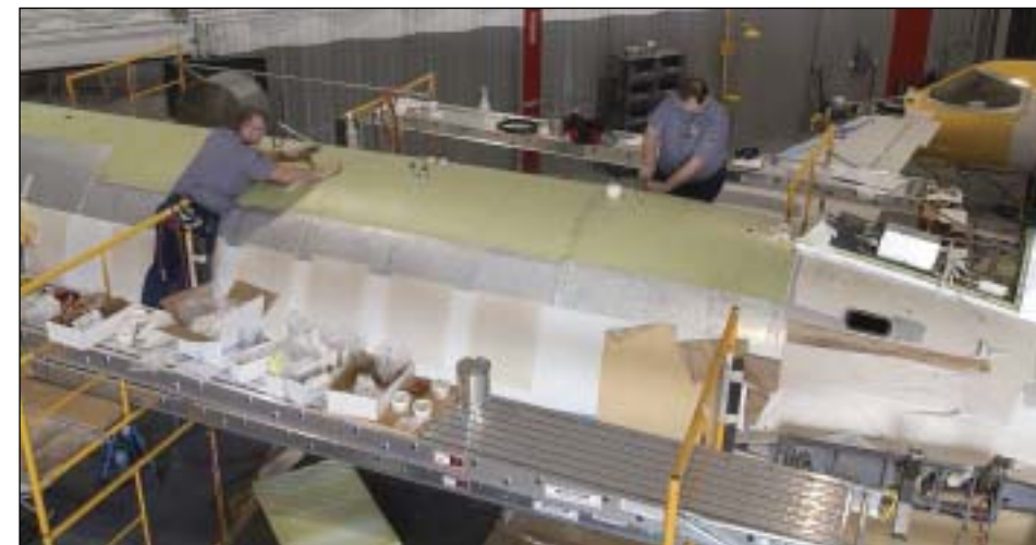
Duncan Aviation’s Structures Technicians replace this Hawker fuselage’s top skin, which was damaged by hail.
